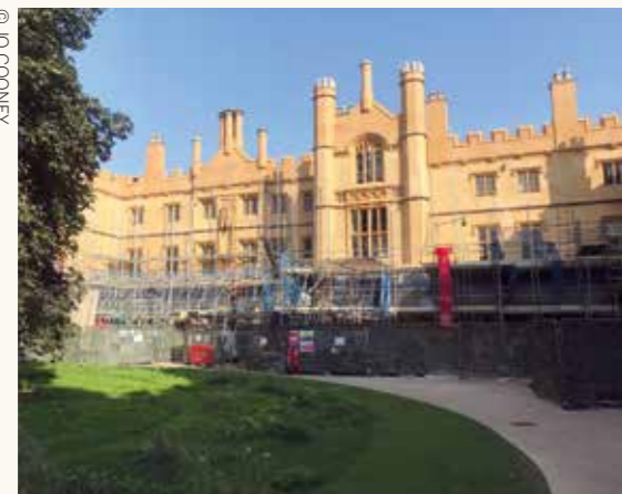
Maintenance work in New Court, summer 2020.
