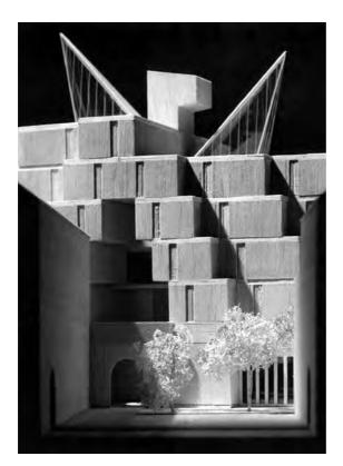
This image shows how Architects' Co-Partnership intended the Wolfson to be finished in vertically ribbed exposed aggregate. They regretted that the College's decision to encase the concrete with horizontal bands of light-coloured brickwork had turned their 'soaring monolith into something more like a pile of boxes staggered one on top of another (see p.147).
