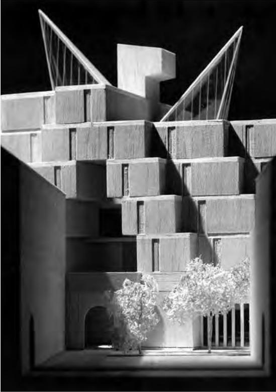
This image shows how Architects' Co-Partnership intended the Wolfson to be finished in vertically ribbed exposed aggregate. They regretted that the College's decision to encase the concrete with horizontal bands of light-coloured brickwork had turned their 'soaring monolith into something more like a pile of boxes staggered one on top of another' (see p.147).
